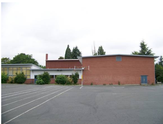
East (side) elevation of the west wing
