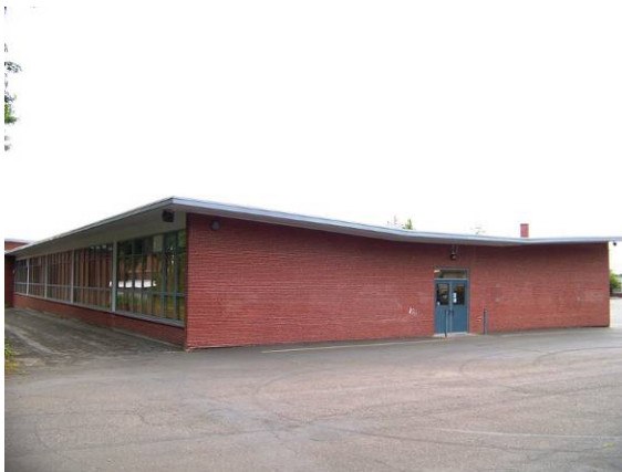
South (rear) and west (side) elevations of the west wing
